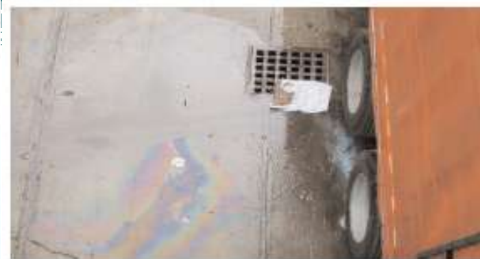
This oil sheen, left by parked vehicles, makes its way towards this catch basin and storm drain network. Without proper treatment, the oil will enter the nearest surface water, where it will degrade fisheries habitats.
